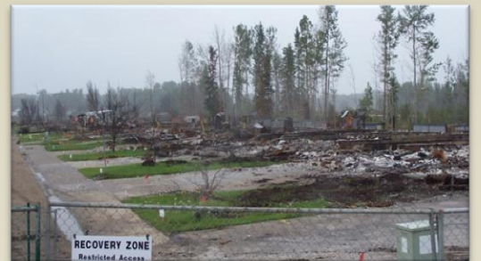
"We had daily meetings with the demolition group – work started early June to mid-September"
