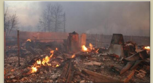
"We needed a methodical demolition to allow methodical construction"
